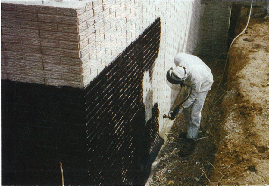
■ When waterproofing products are properly applied, it is possible to keep moisture out of the structure for 30 years or more.
